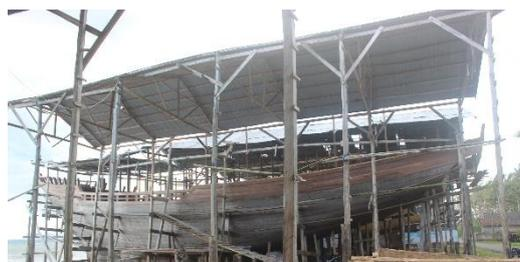
**Figure 1.** Phinisi ship manufacturing process
